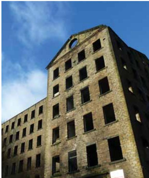
3.45 The mill is of six storeys plus attic and is arranged in an L-Plan. It has 15 x 5 bays with a further 4 bay wing to the right. The mill is the oldest and largest surviving example of a multi-storey, steam powered, iron framed textile mill in the important textile centre of Halifax. Old Lane Mill's attached boiler house and chimney are listed separately from the main mill building. They are also listed Grade II\*.
